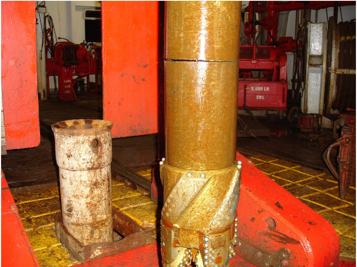
Figure F69. Bit sub under tension on the rotary table. Note the large crack that extends most of the way around the circumference.
