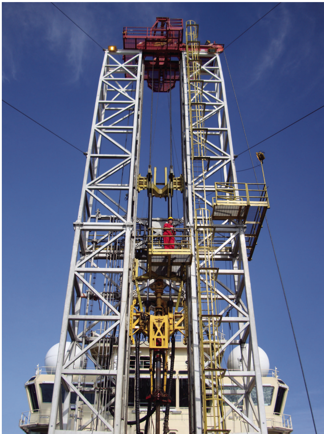
Figure F5. Bluestone TT150 derrick showing the rooster box from which downhole logging operations were conducted during Expedition 325. (Image courtesy of D.Smith@ECORD_IODP.)
