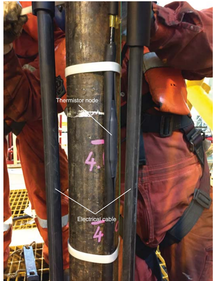
Figure F15. Spacing of centralizers, tie wraps, and steel bands used to secure cables to 3½ inch tubing, Hole C0010A. FWD = forward.
