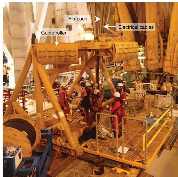
Figure F10. Guide roller over the moonpool used to support tubing and cables during deployment, Hole C0010A.
