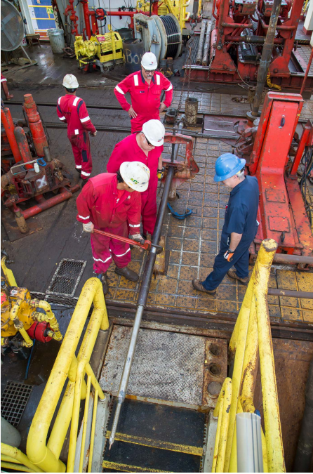
Figure F9. Final preparations for the WSTP were conducted on the rig floor prior to deployment within the cased borehole.
